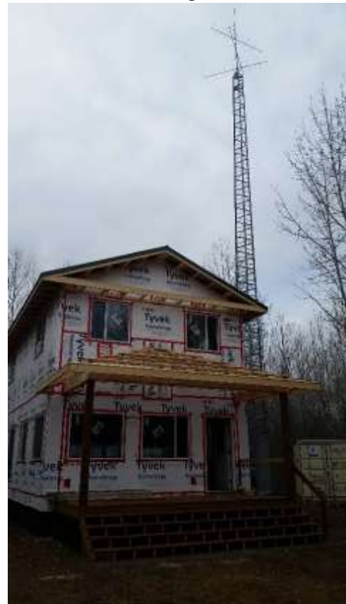
Our new education and research station under construction
